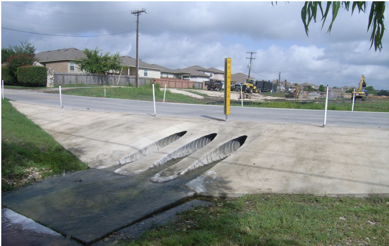
Figure 5: Klein Road Existing Low Water Crossing
