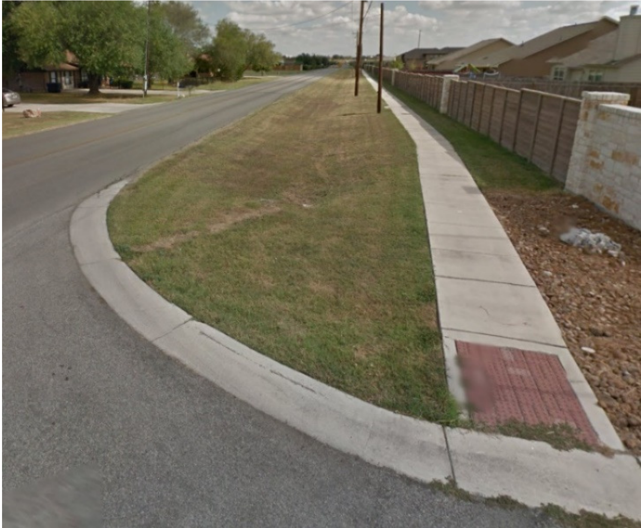
Figure 1: Klein Road Existing Pedestrian Facilities
